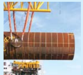
All 140 turbine foundation monopiles were installed using the first set of lifting slings. After completion Lloyd's proof loaded the slings and recertified them for continued use.
