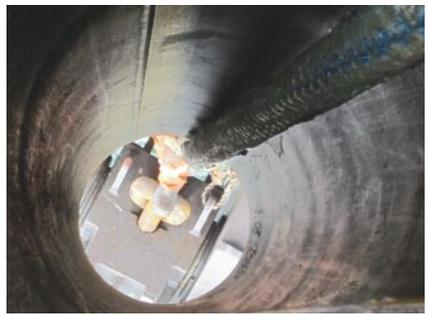
*A view of the anchor-chain tensioning down the internal cavity of the I-tube.*
