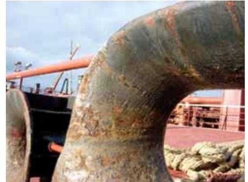
*Rust damaged chock typical of crude tankers.*
