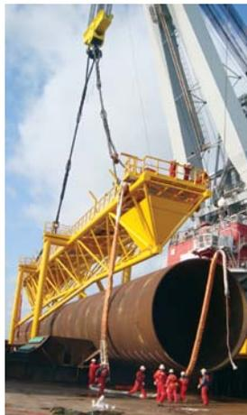
By the end of the third quarter of 2010, all 140 turbine foundation monopiles were installed using the first set of lifting slings.
