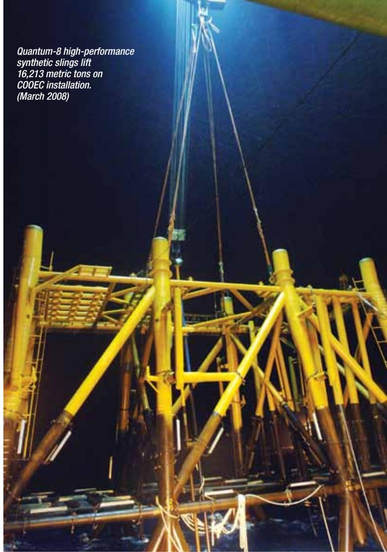
COOEC reports that the slings outperformed either the cable-laid wire or the synthetic webbing slings they had been using. The lightweight, easy handling Quantum-8 slings were attached manually, without the assistance of heavy equipment required by cable-laid or synthetic webbing alternatives, resulting in a faster, more efficient installation.
