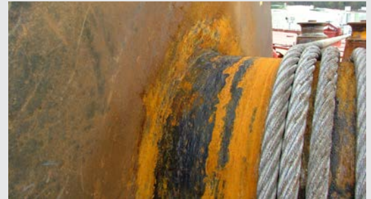
Winch drums and flanges should be free of rust, corrosion and scoring damage from wire rope before HMPE mooring lines are installed.
