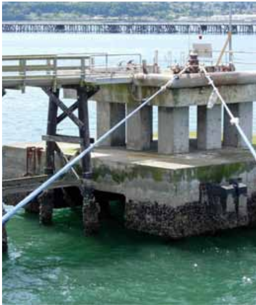
Mooring lines with twist induced.
